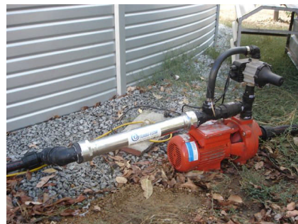
Model T220 Turbu-Flow On Irrigation Pump
