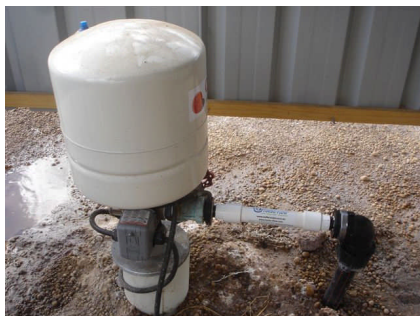
Model T34D Turbu-Flow On Bore Pump
